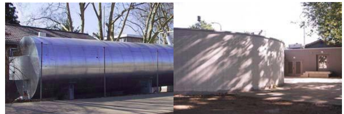
Figure 2. Plug-flow digester followed by stirred after-digester for the digestion of organic materials at the zoo in Heidelberg [5]
